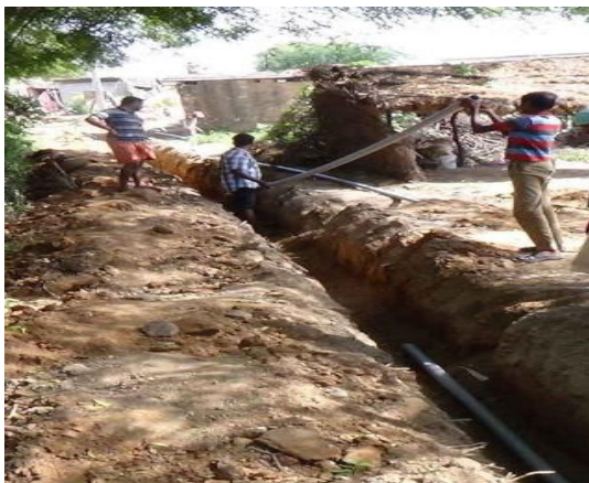
Figure 13 Reinstalling Faulty Water Distribution Pipes
